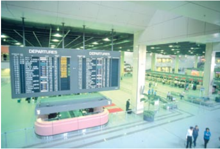
Commercial air conditioning is used in modern airports, hospitals, and other commercial facilities.
